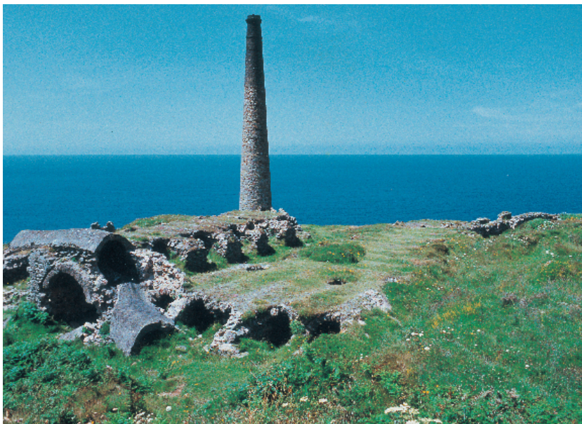
Plate 8a. Arsenic calciner, Botallack Mine [SW 3641 3322] (Photograph © A.J.J. Goode) Arsenic ores were roasted in the Brunton calciner and the resultant arsenical fumes were condensed in a 'labyrinth'
