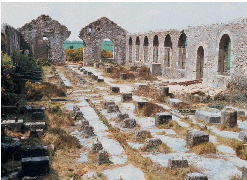
Plate 8b. Dressing floors, Wheal Basset, Vanner House [SW 6910 3990] (Photograph © A.J.J. Goode). Lighter fractions of the crushed ores were washed away here, leaving heavy concentrate
